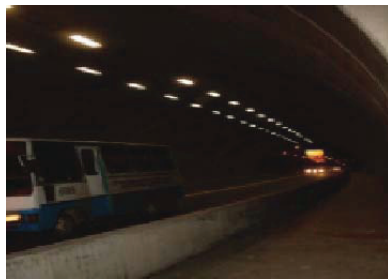
Figure 10: Tunnel used for preliminary testing
